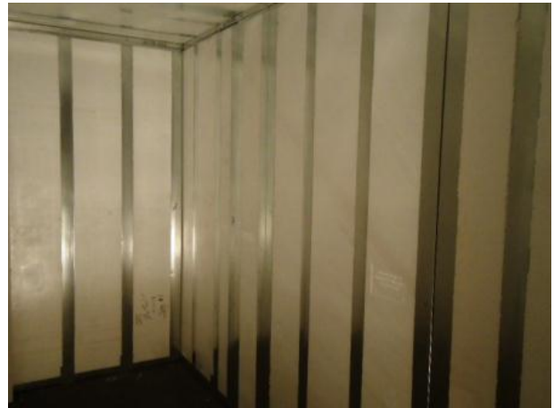
Before Gypsum Board
